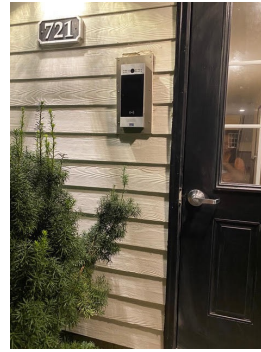
(Satin Aluminum Plate on a PVC board that we mounted into the wall)
